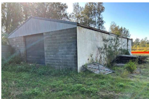
Looking north-east showing the existing shed in the north-west corner of the site. The shed is of masonry block construction on a concrete slab with a corrugated metal roof.
